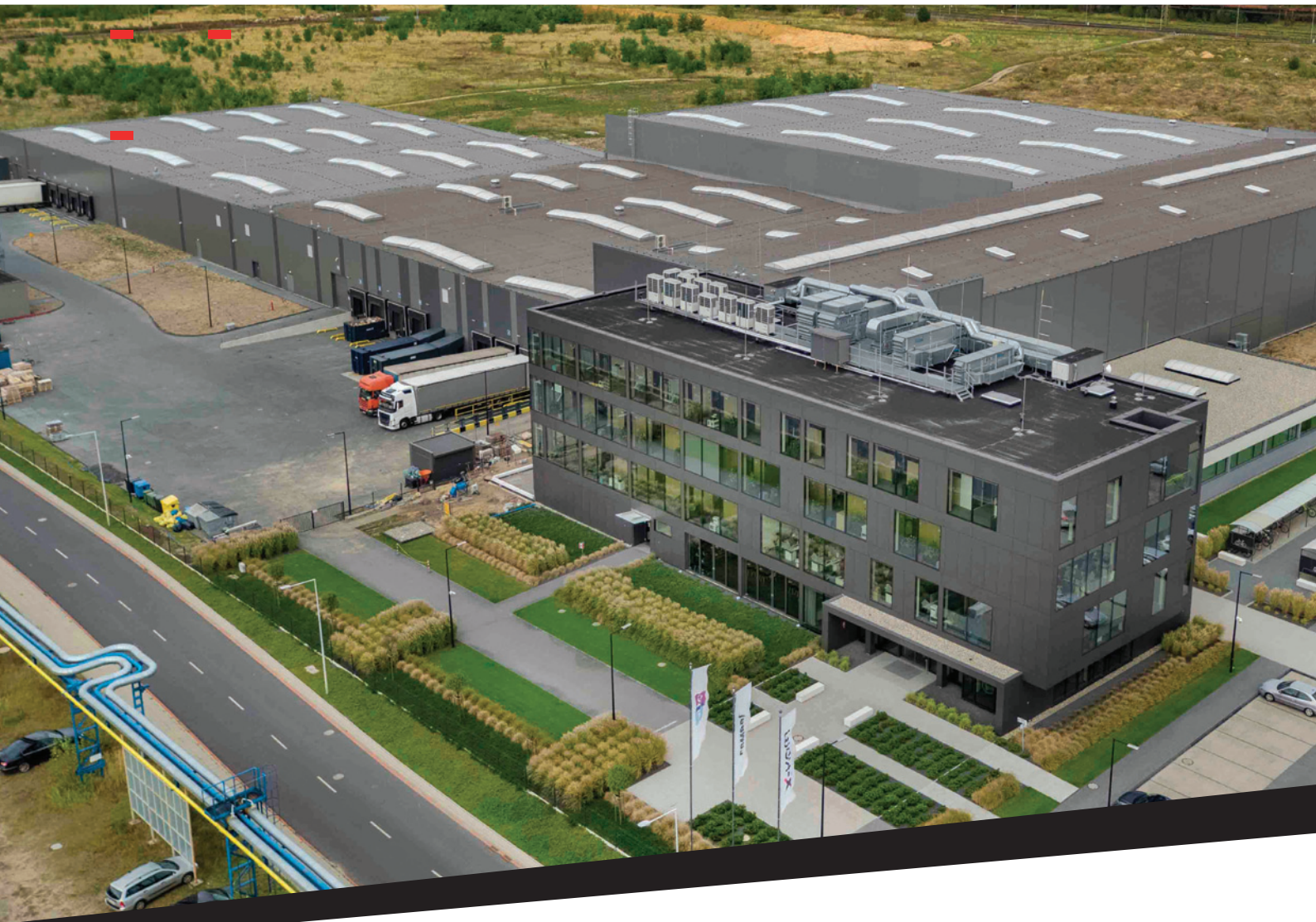
Warehouse hall, office and production building, pumping station, x-kom (Częstochowa)
